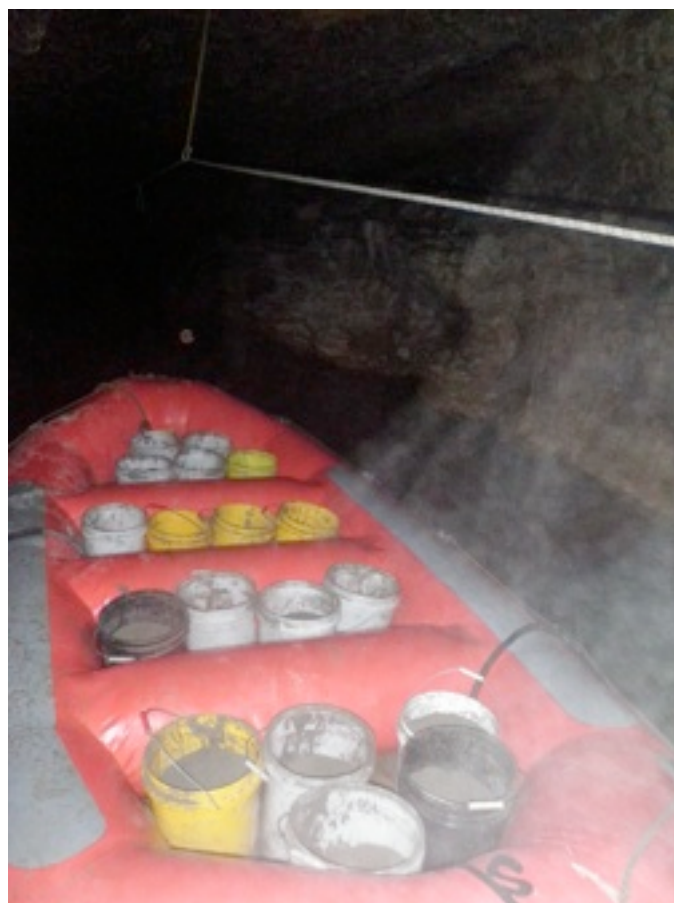
Red raft put to use transporting concrete
