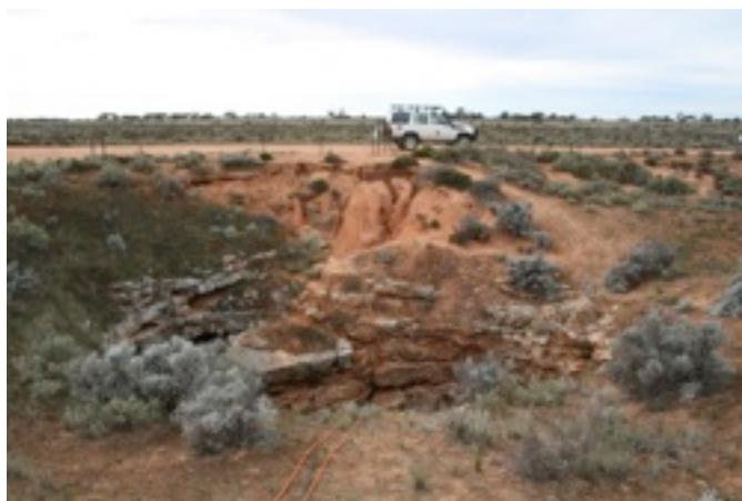
Nullarbor erosion issues. Pannikin Cave, Western Australia 2009.
