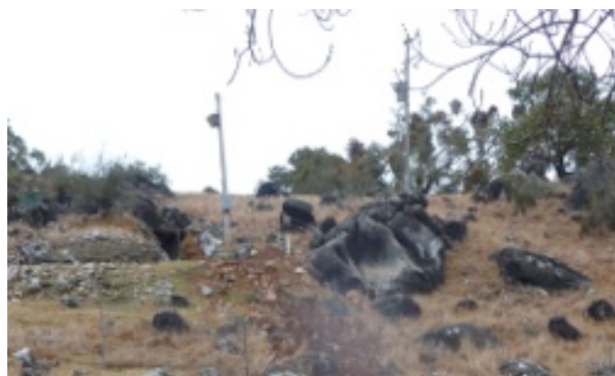
Right. Power pole prior to the new work
